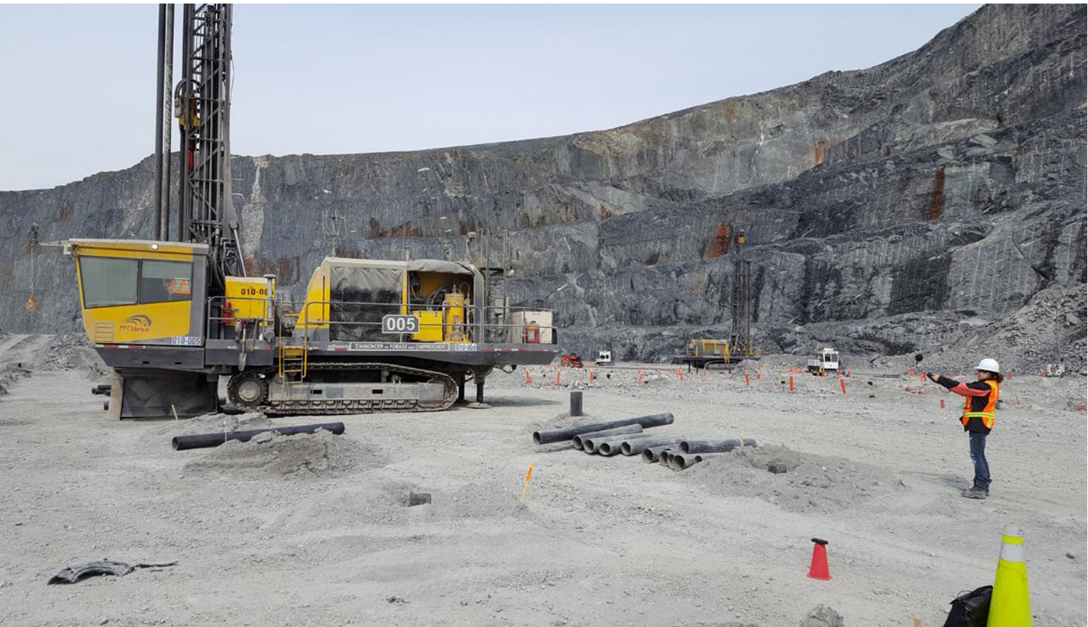
▲ Noise measurements on a Pit Viper drill using a Concerto portable device
