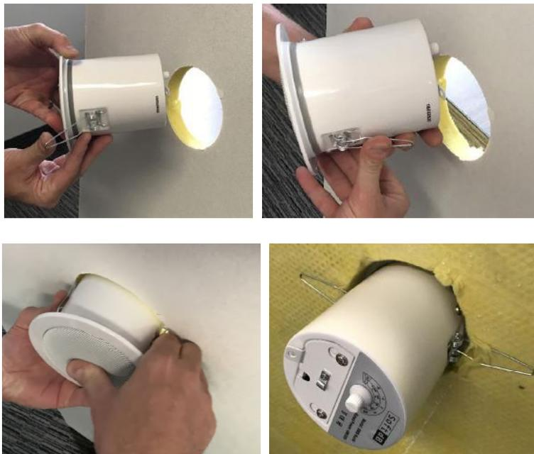
*Note: If the local regulations require an anchor, use the small ring on the back of the speaker to hang a safety chain.*
